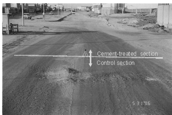
FIG. 1—Comparison of pavement status for cement treated calcareous base course section and a section with untreated calcareous base course.
